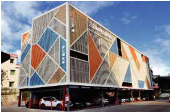
Dongguan Sanyuanli Financial Street (Phase I) Address: East of Zhongji Caijin Business Building, Guantai Road, Dongguan City Equipment Type: Six-level Lifting and Traversing Parking System
