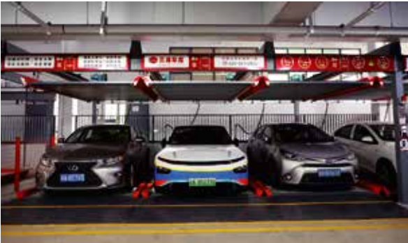
Trial Business Building of Guangzhou Railway Transportation Court Address: No. 48 Xinhua Road, Xinhua Town, Huadu District, Guangzhou City Equipment Type: Two-level Lifting and Traversing Parking System
