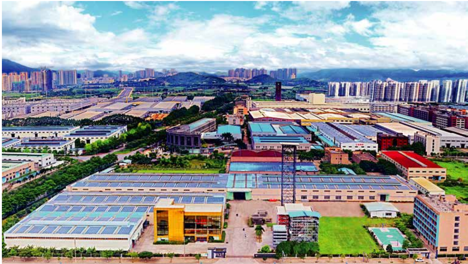
Sampu Domestic Intelligent Manufacturing Base
